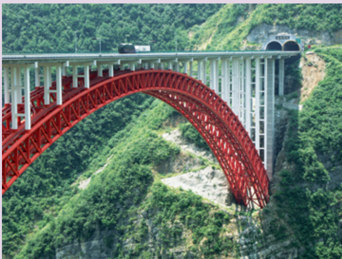
Location of the both parallel steel arches.
