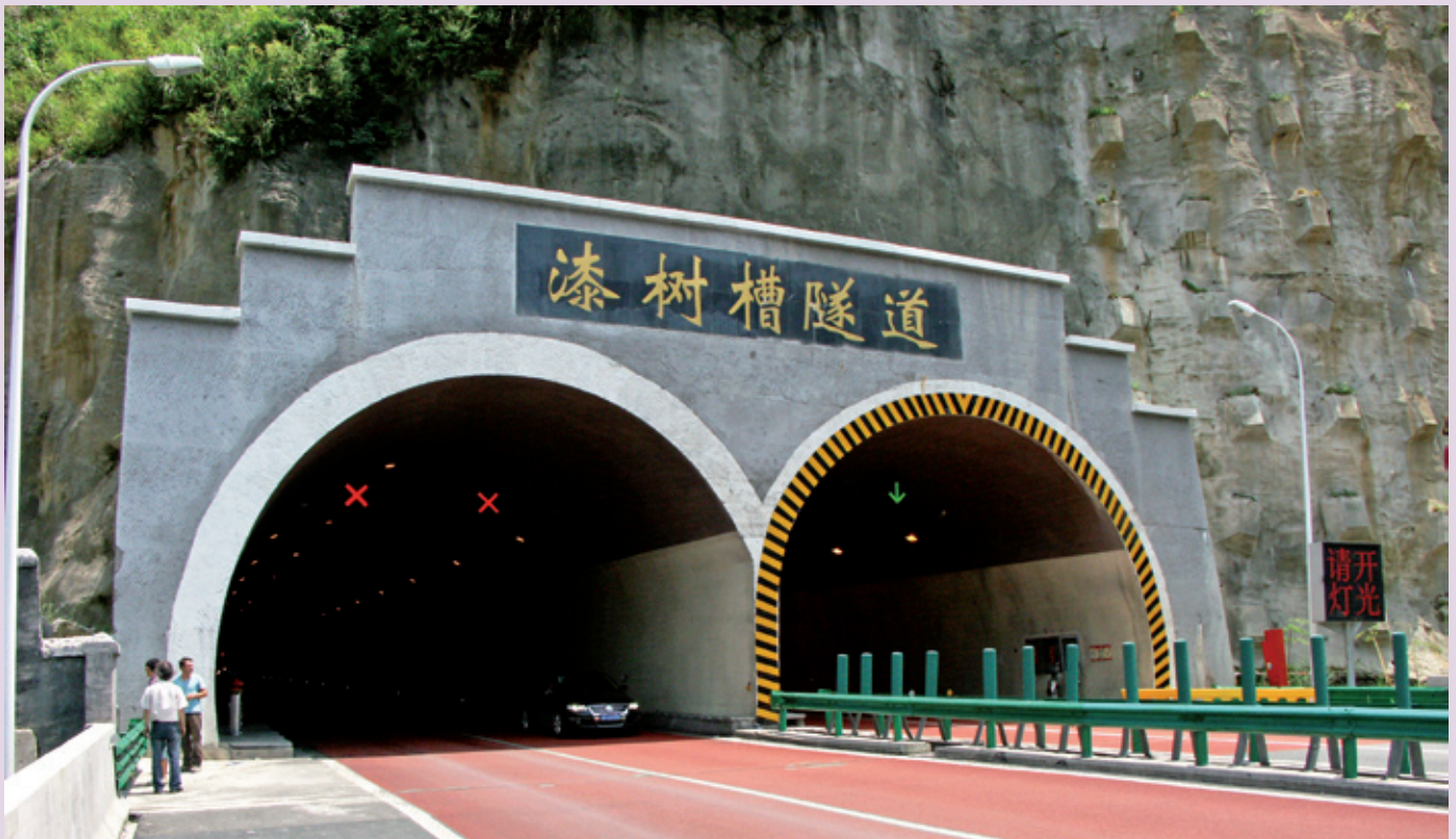
Tunnels at the west end of the bridge.
