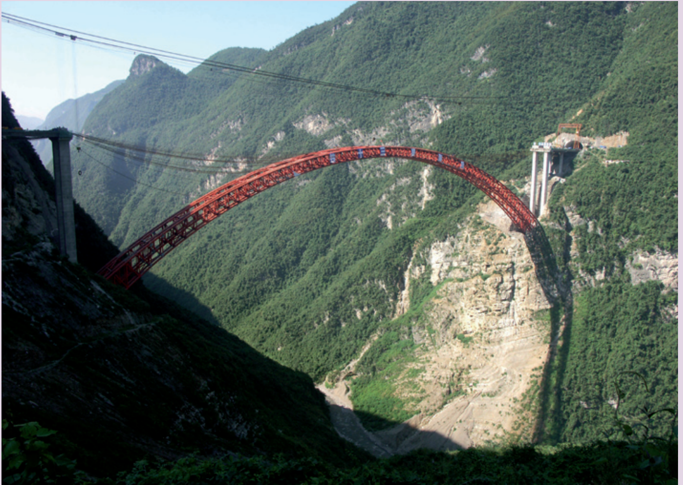
The first arch under construction.
